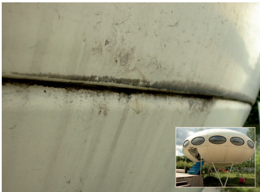
Fig 4 | Futuro , designed in 1965 by Matti Suuronen, showing evidence of microbial growth. Images courtesy of Tim Bechthold (Museum Die Neue Sammlung, Munich, Germany) and Francesca Cappitelli (Cappitelli et al , 2006b). Reprinted with permission from Elsevier.
