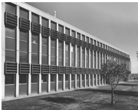
The now demolished Research Laboratories designed by Harry Norris and Associates constructed in 1962–63 Photograph by Wolfgang Sievers Courtesy of the National Library of Australia
