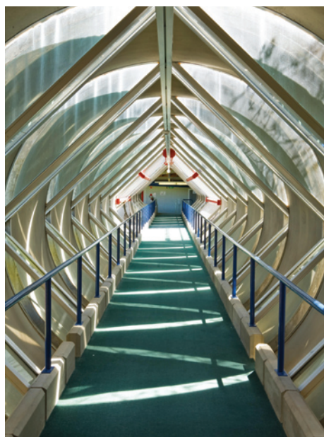
Clyde Cameron College, Wodonga (Kevin Borland) Photograph by Heritage Victoria
