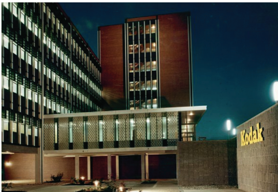
The nearly completed Administrative Building in 1962 Photograph by Wolfgang Sievers Courtesy of the National Library of Australia
