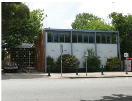
The former Benalla Shire Offices, 2009 Photographer Conrad Hamann
