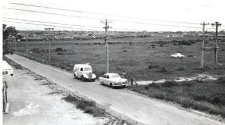
Surveying the 'greenfields' Kodak site viewed across an unmade Elizabeth St, circa 1954. Source: Kodak Australasia
