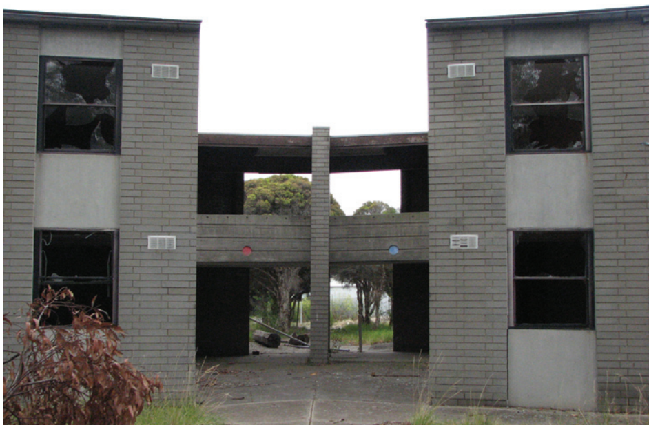
Detail of crossover (Phillip Hostel)
