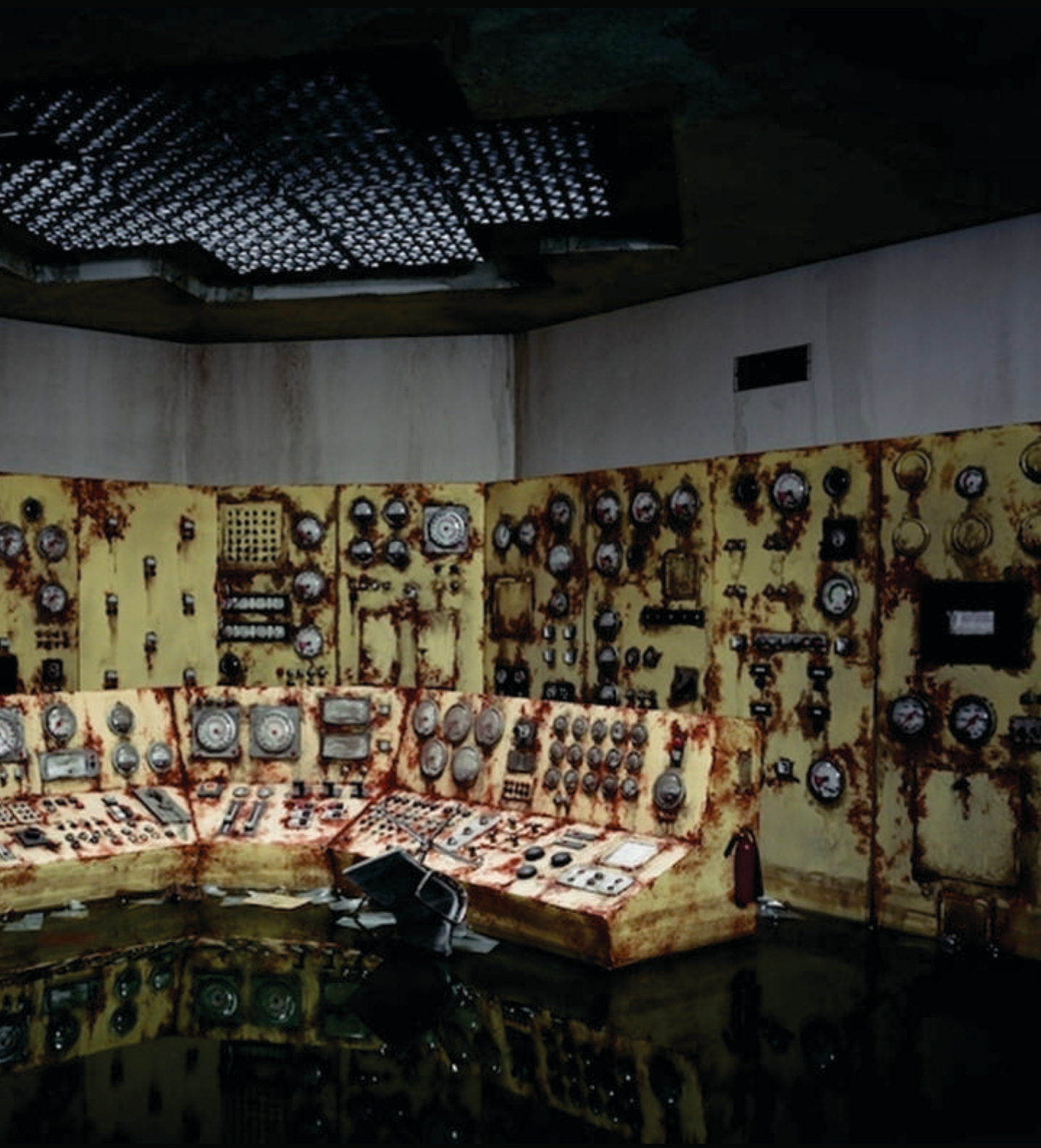
Lory Nix, Control Room 2010.
