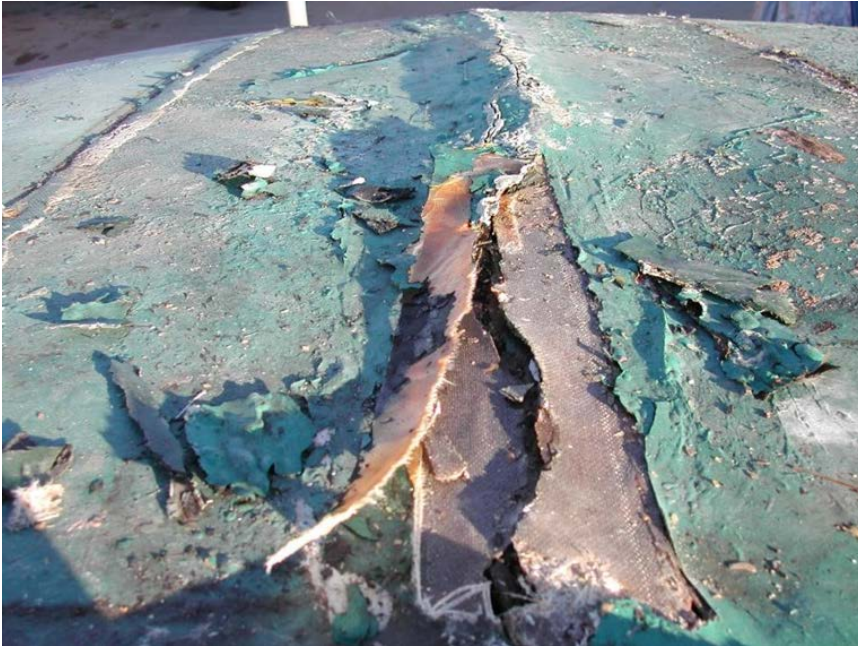
Figure 10 Near top of door opening where upper and lower halves of shell are joined; vertical joint is connected with steel bolts, December 2002. Source: Milford Wayne Donaldson, FAIA.
