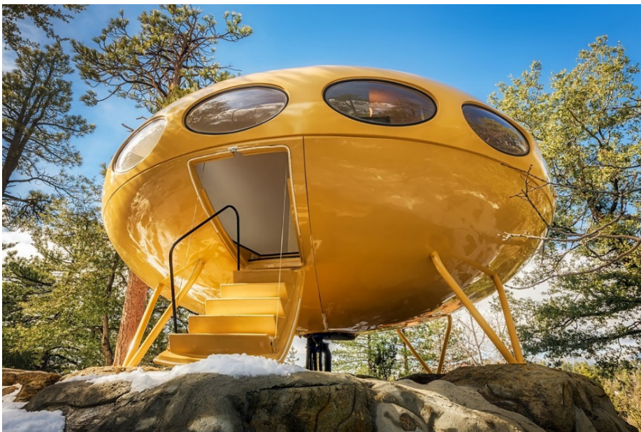
Photo 7 Hinged downward opening door and integral stairs similar to a Cessna Citation aircraft, camera facing northwest
