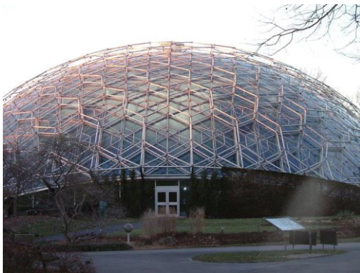
The Climatron greenhouse at Missouri Botanical Gardens (1960) Architect Thomas C. Howard
