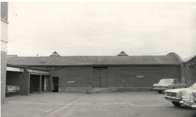
Porter Prefabricated Iron Store (Assembled)
